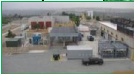
3.2 MW Landfill Gas Energy Plant
